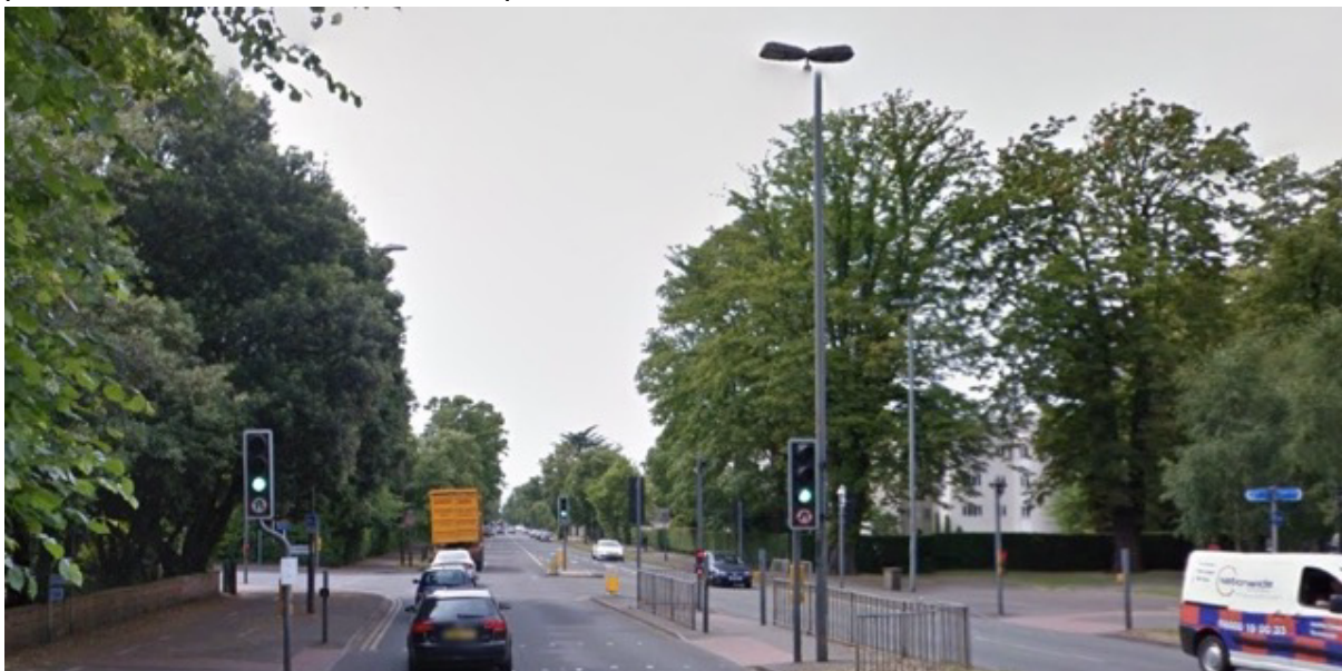
pedestrian and cycle crossing at junction of Lansdown Road, Hatherley Road and Queens Road. Pedestrians and cyclists are corralled into a narrow fenced off area and have to cross on two phases of lights.
